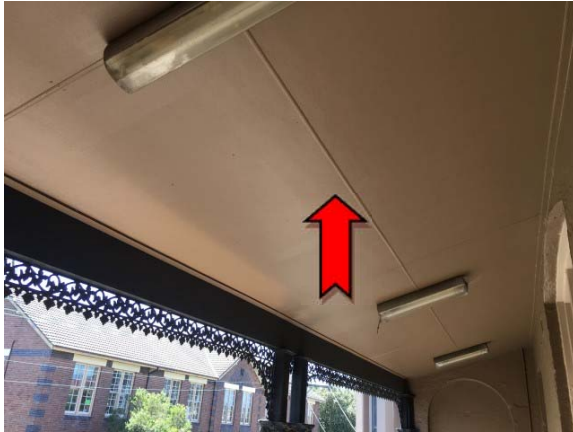
Photo 1. Exterior, level one, verandah, awning – suspected asbestos-containing fibre cement sheeting.
